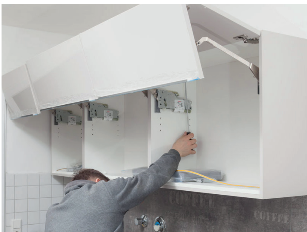
Fastening wall cabinets
