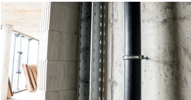
Fastening of cable ducts
