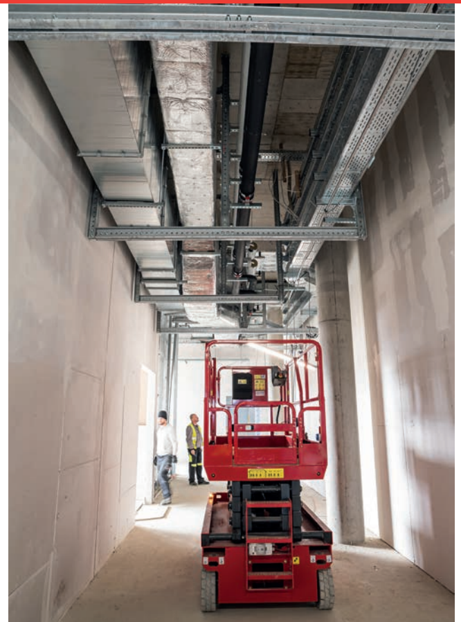
Fastening ventilation ducts
