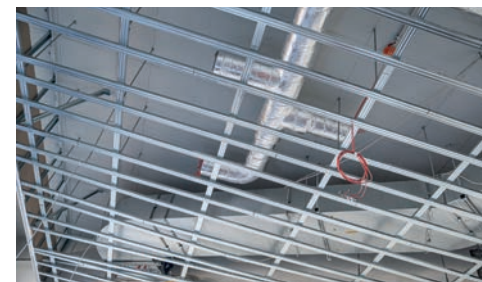
Fastening ventilation ducts
