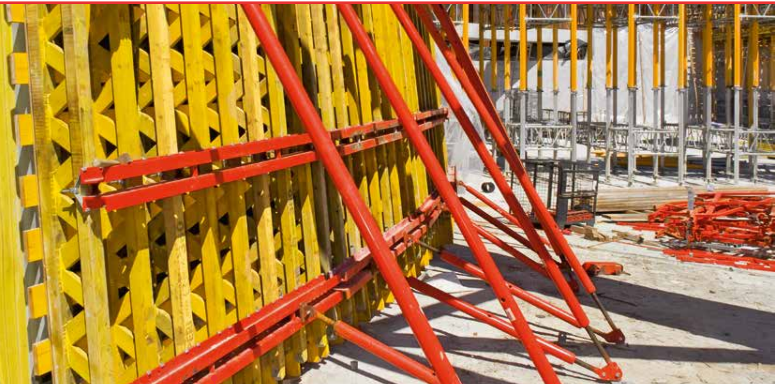
Fastening of guardrails, scaffolding or formwork props
