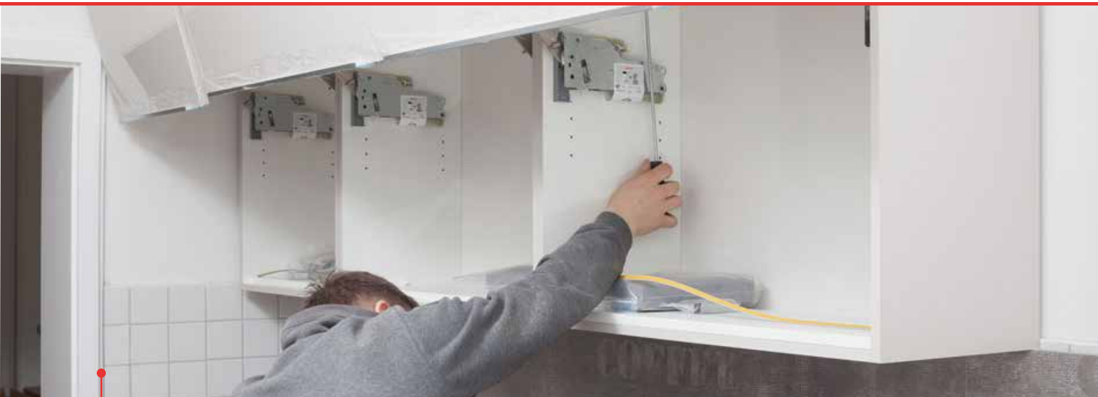
Fastening wall cabinets
