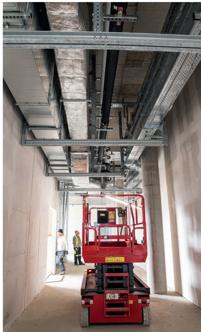
Fastening of ceiling suspension of any kind
