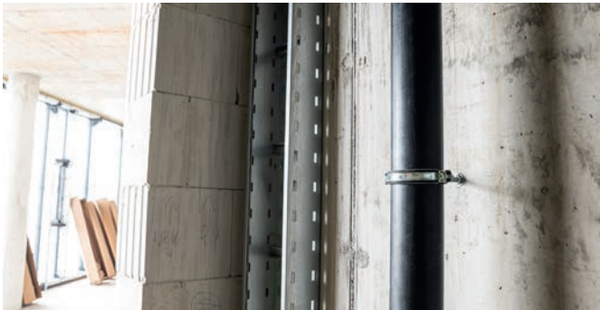
Fastening of cable ducts
