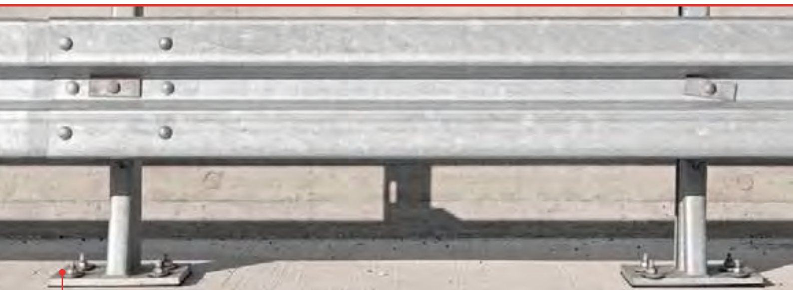
Fastening of crash barrier systems
