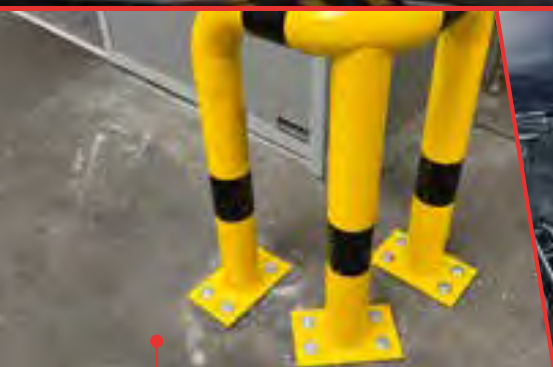
Fastening of impact protection systems
