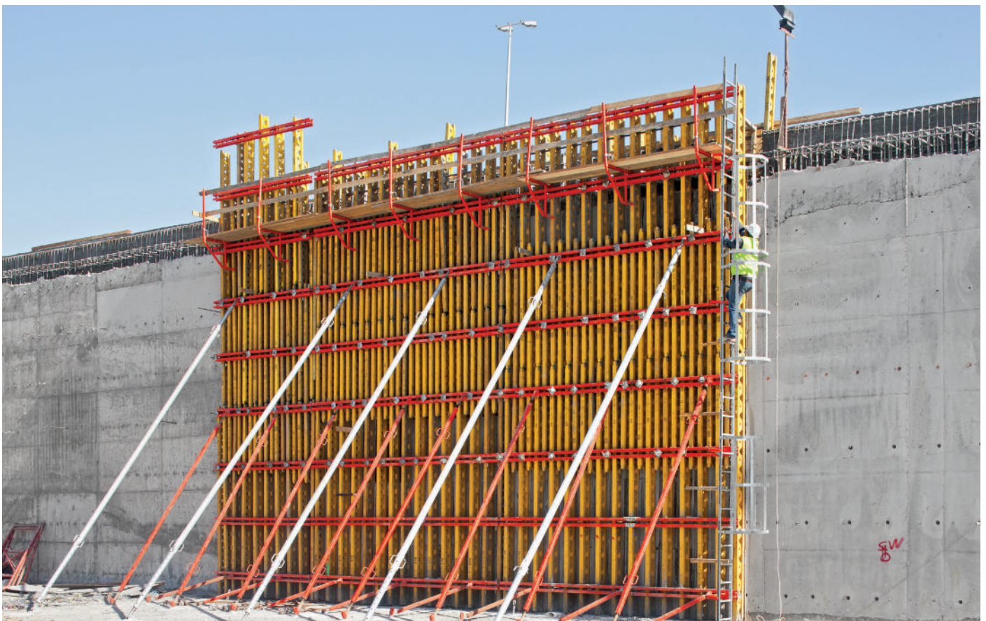
Fastening of guardrails, scaffolding or formwork props
