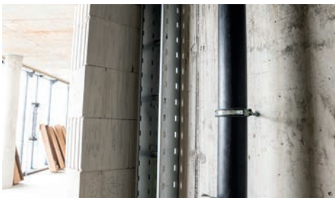
Fastening cable ducts
