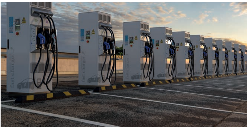
Fastening of e-charging columns
