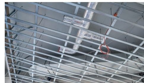
Fastening ventilation ducts
