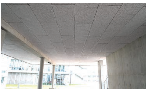
Underground parking and basement ceilings
