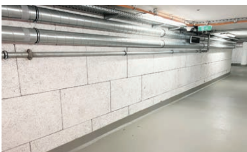
Underground garage and basement walls
