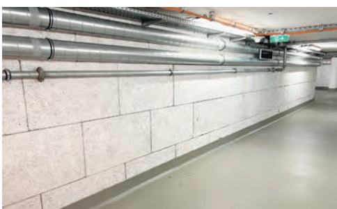
Underground garage and basement walls
