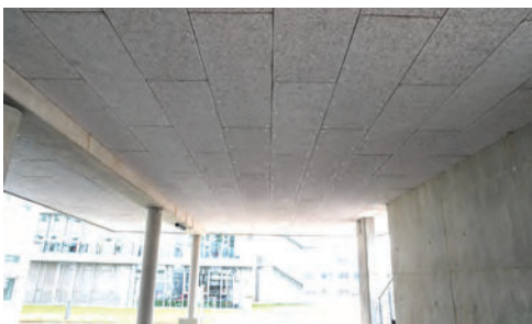
Underground parking and basement ceilings
