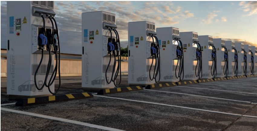
Fastening of e-charging columns
