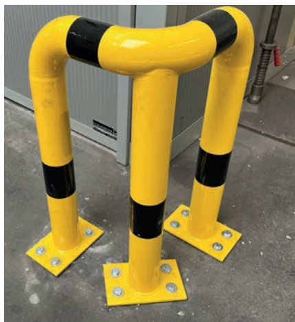
Fastening of impact protection systems
