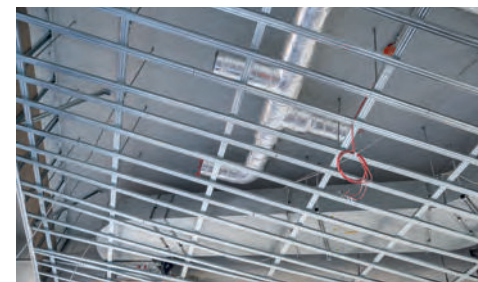
Fastening ventilation ducts
