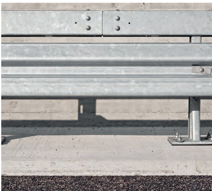
Fastening of crash barrier systems
