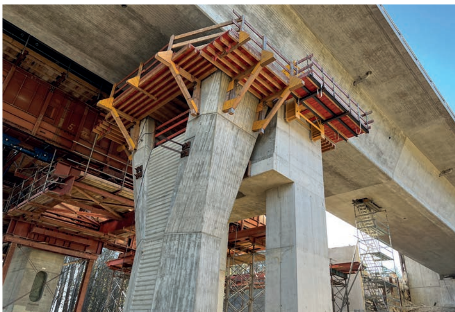
Fixing scaffolding and formwork in the renovation area
